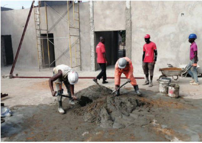
Work in progress on the community centre
